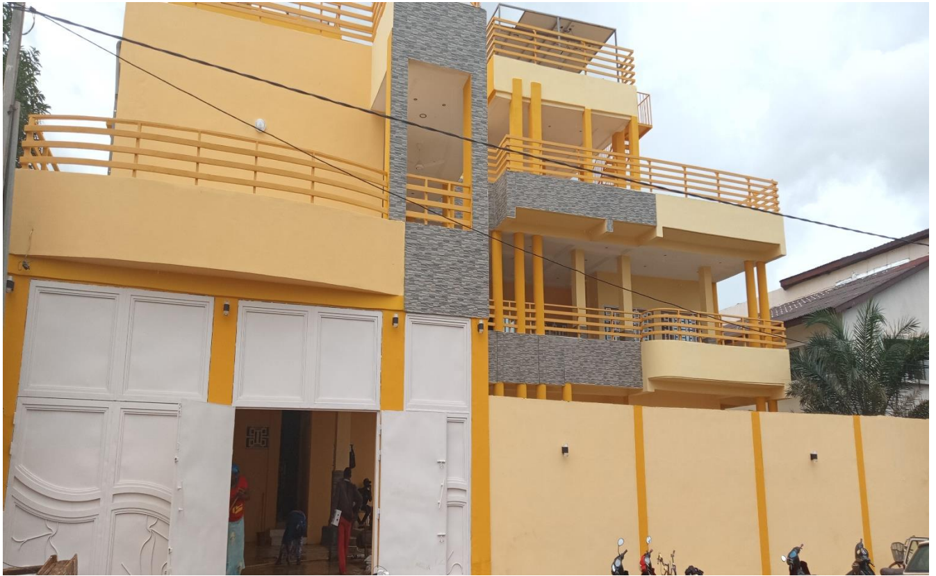
Figure 2: Presentation du chantier
