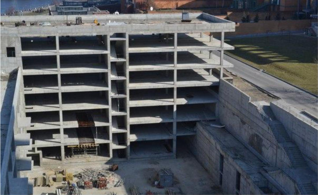
Civil 7 floors building with underground parking Dnipropetrovsk Ukraine 2013
